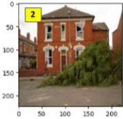
Many trees had fallen and, a building was damaged.
